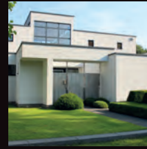
Find insulation problems
